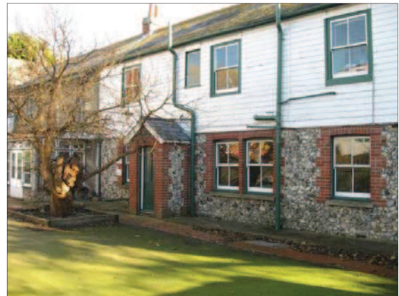
Curtilage listed terraced cottages
