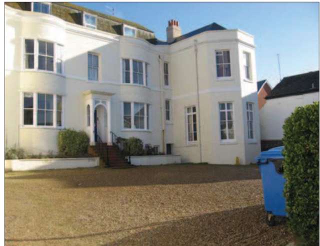
Small car parking area
